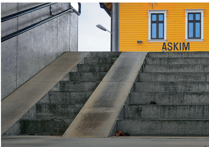
Figure 2.6: Specially designed ramp
